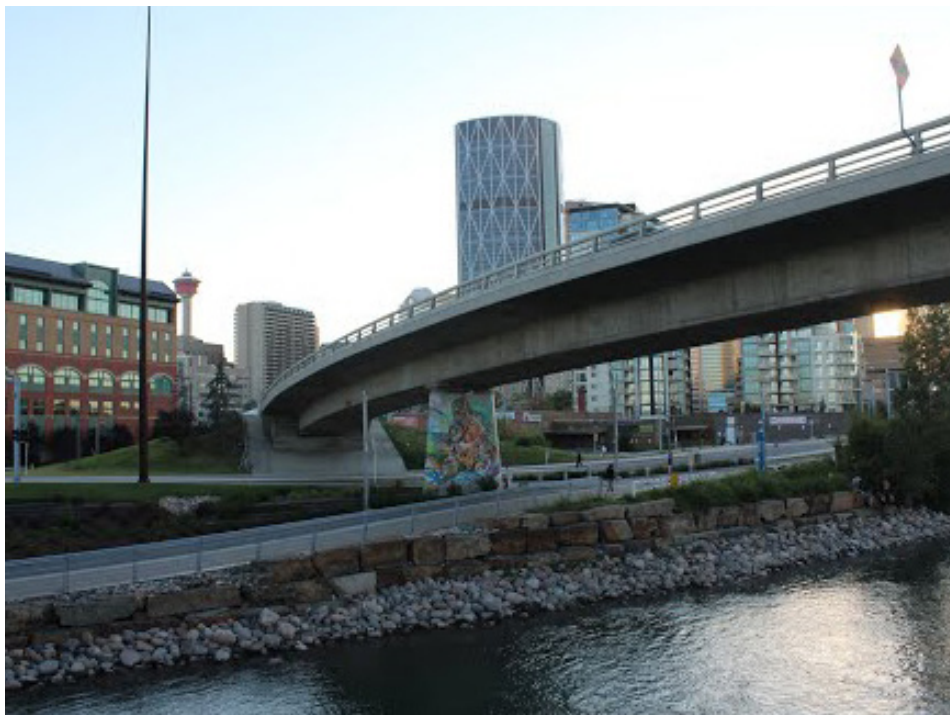
View of the project site
