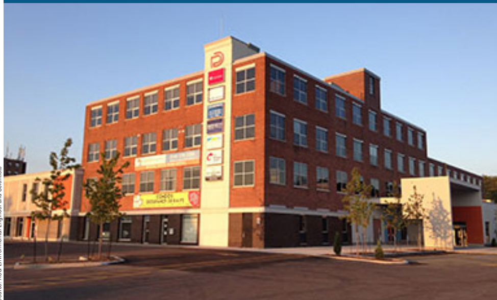
Exterior of Centre Suites.
