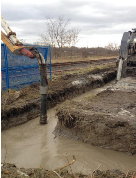
An installation of an on-site concrete barrier, to prevent against the potential future migration of off-site contaminants.
