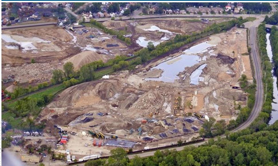
Aerial view of site during remediation.
