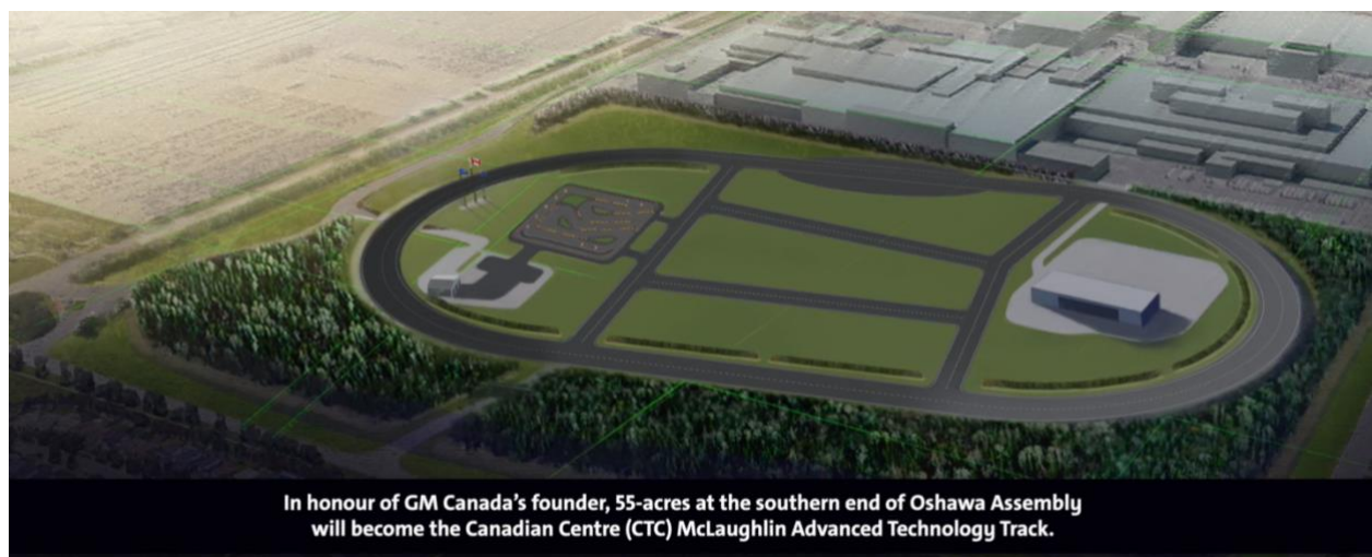
Figure 10 – A screenshot from GM Canada's website displays the future AV Testing Track at its former plant in Oshawa. This 55-acre track will be located on the south of the site and will allow research and development to continue in Oshawa.
