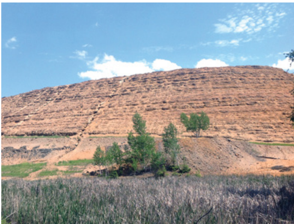
Area B, the tallest waste pile on site, was leveled and moved to Area C during the early stages of remediation.
