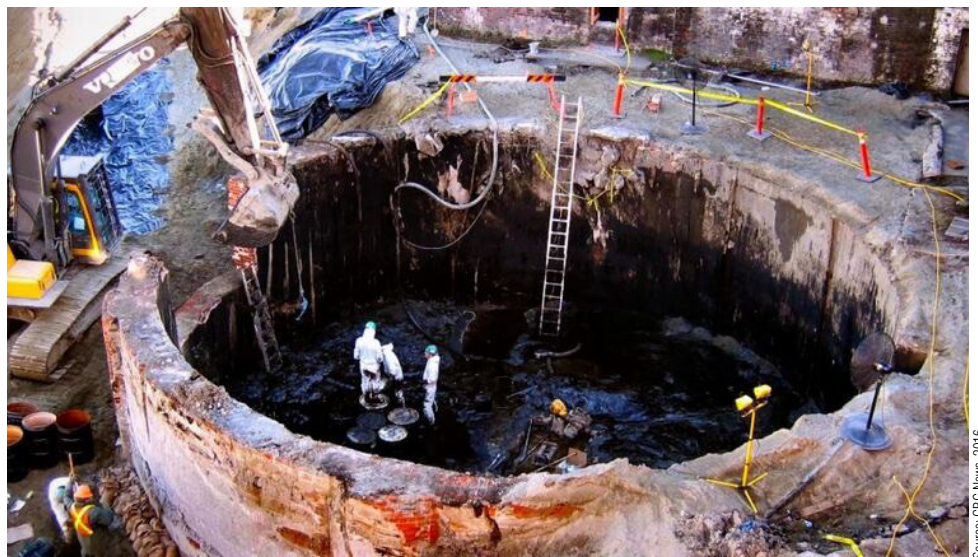
Figure 3. Photo of tar well excavation and clean up process
