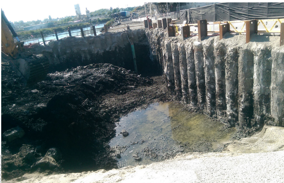
Figure 4. Photo of excavation within the newly installed secant barrier walls
