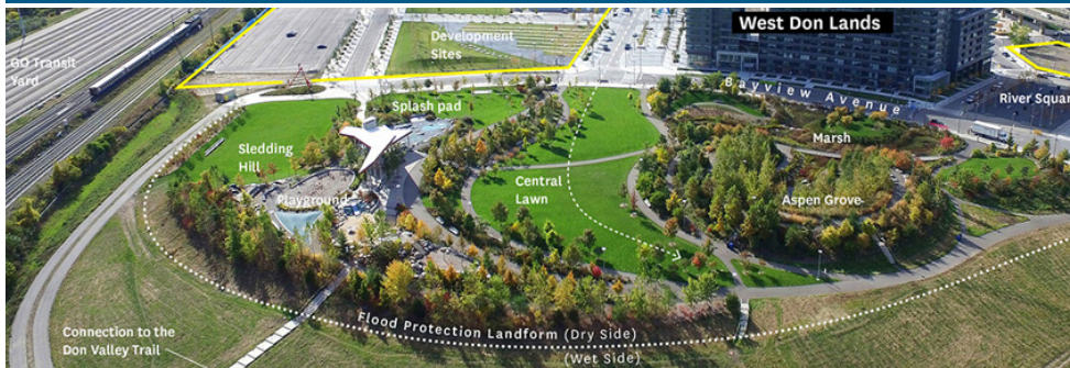
Figure 1: An aerial image of the complete Corktown Common project at full build out
