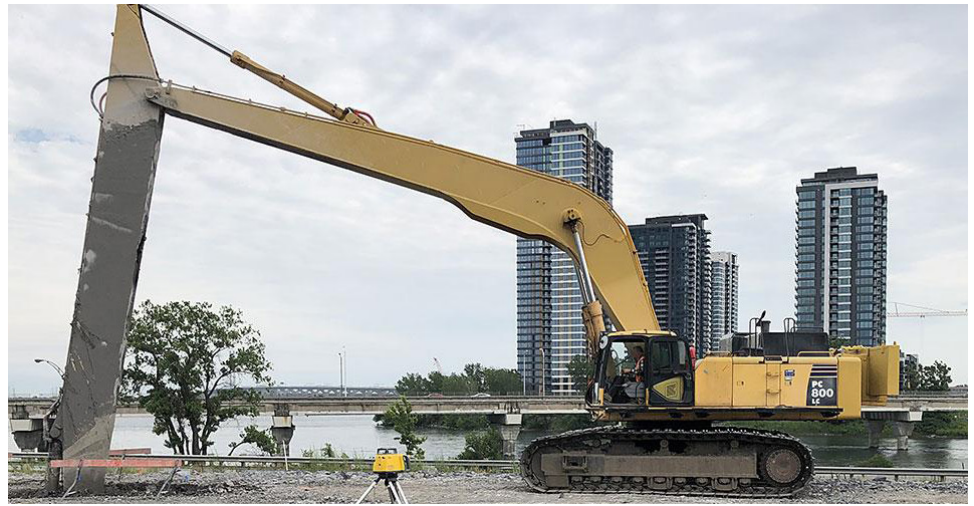
Site preparation for slurry wall and collector installation.
