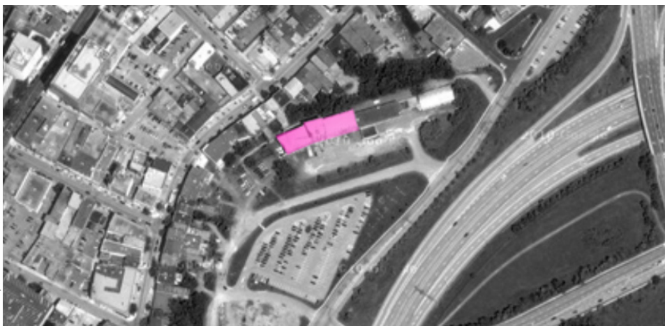
Aerial Photos (1934 above, 2010 below) of the property, illustrating the changing infrastructure in St. Catharines. 198 St. Paul street was originally situated next to the first and second Welland Canal, now Hwy. 406.
