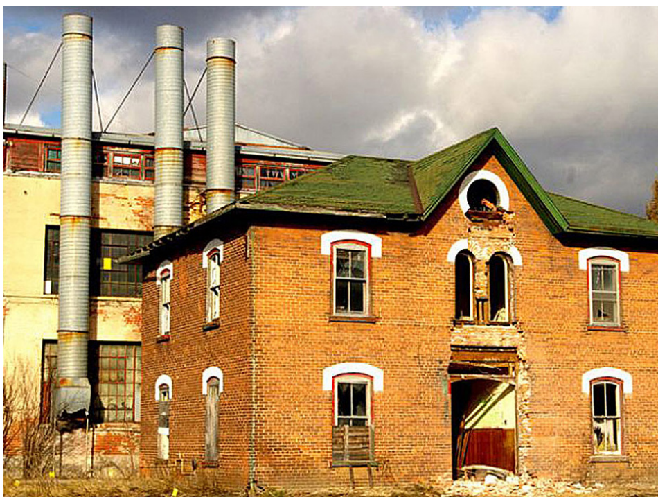
A derelict Tannery Factory existed on the site prior to its demolition in 2007.
